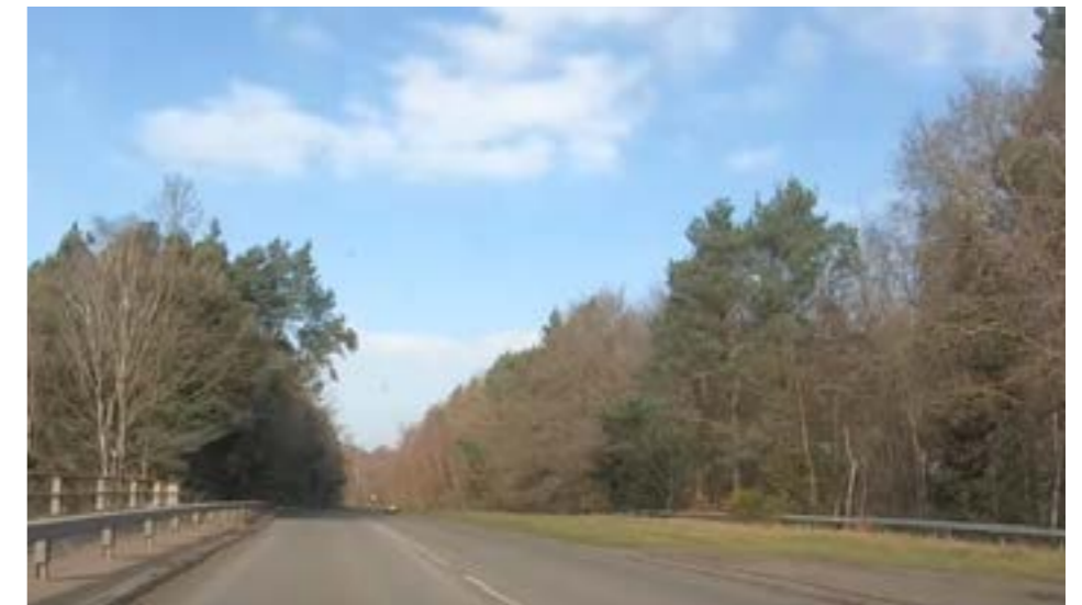
Minley Road M3 overpass
