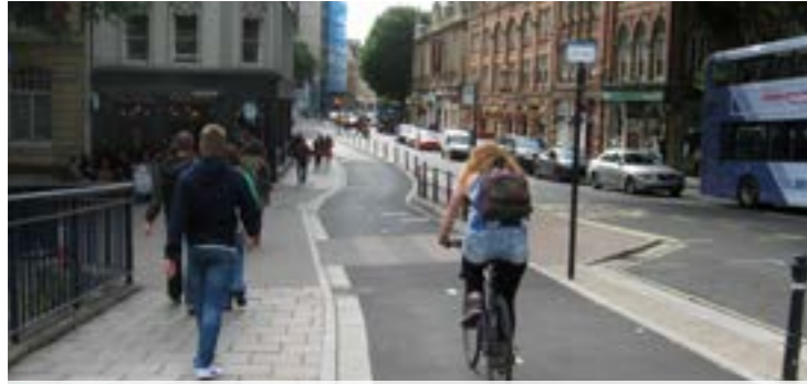
Fully kerbed segregated cycle track
